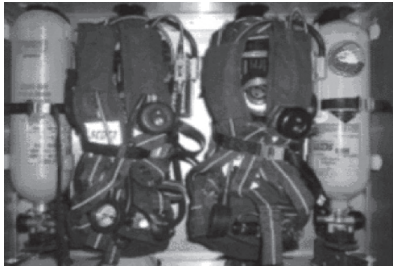
Figure E-1. Locker Designs Often Alternate Between SCBA and a Spare Cylinder of a Different Size
